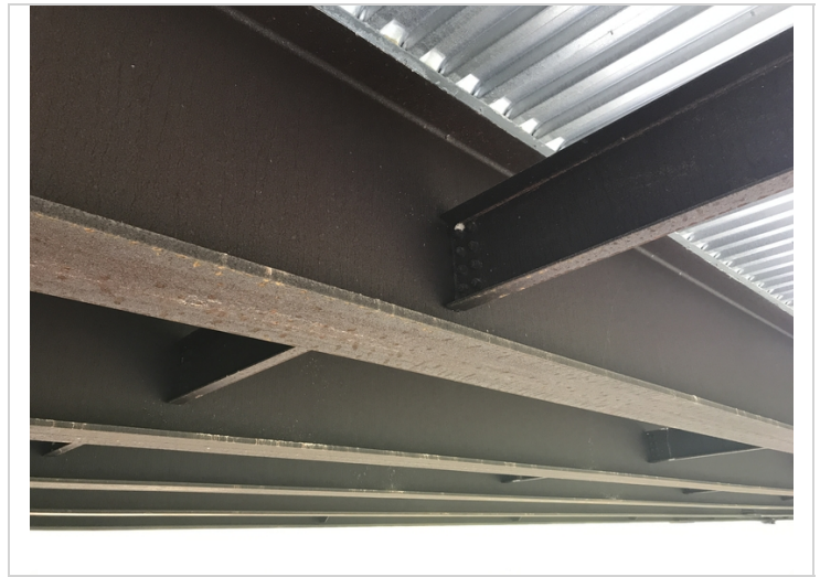
Weathering steel beams
