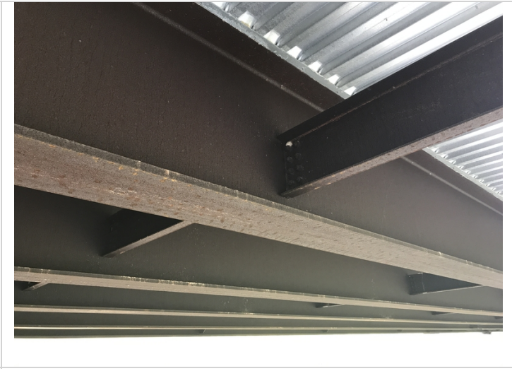
Weathering steel beams
