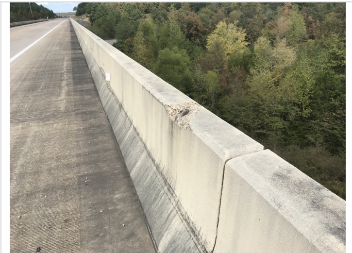
Spall Span #2 Parapet rail
