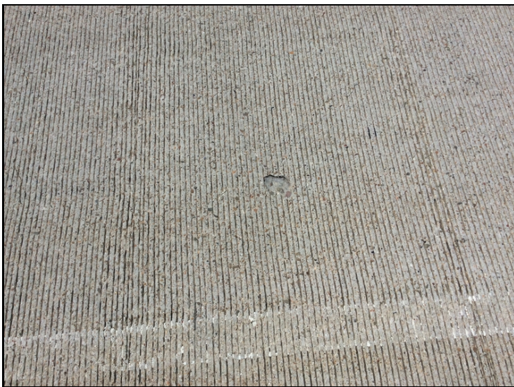
Pop out in deck span 2 north bound lane
