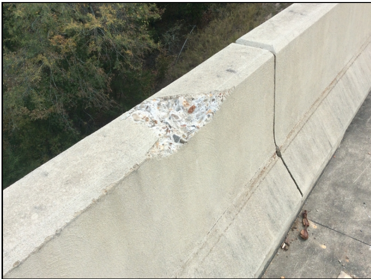
Parapet rail spall span 2 right side
